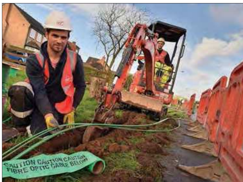
Virgin Media Project Lightning engineers lay fibre optic cable (Image: Virgin Media)
