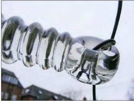
Fig.9. A good aerial is vital. A horizontal loop around the picture rail in a Victorian house is good enough to get the crystal set working, but for best results string it up outside as high and long as possible using glass insulators. I found this insulator on the side of a disused railway!
