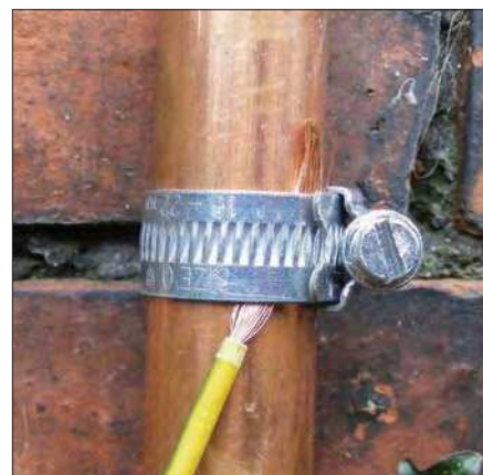
Fig.8. A good earth is needed for a crystal set aerial. Copper water pipes going into the ground are ideal. (Watch out, blue plastic Alkathene pipes are often used for water mains today). Put a steel reinforcing rod into the copper earth pipe if you are going to bang it into hard soil. I used a radiator water pipe as a kid.
