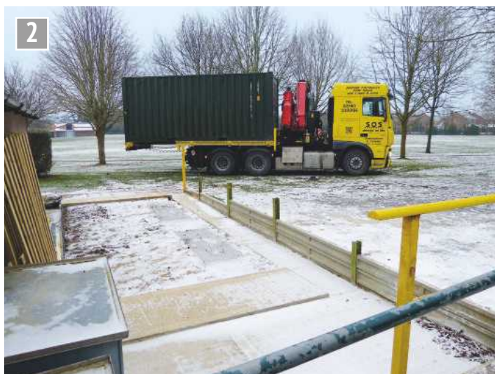
The prepared site showing the concrete pads to take the load. (Photo John Hoyle.)
