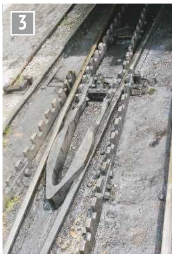
The moving part of the rack at a set of points.
