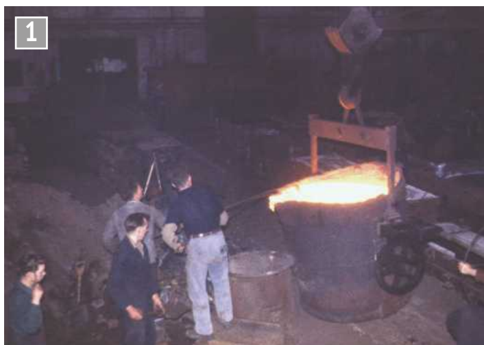
Ladle positioned to pour.
