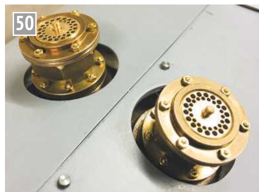
The safety valves mounted on the boiler.
