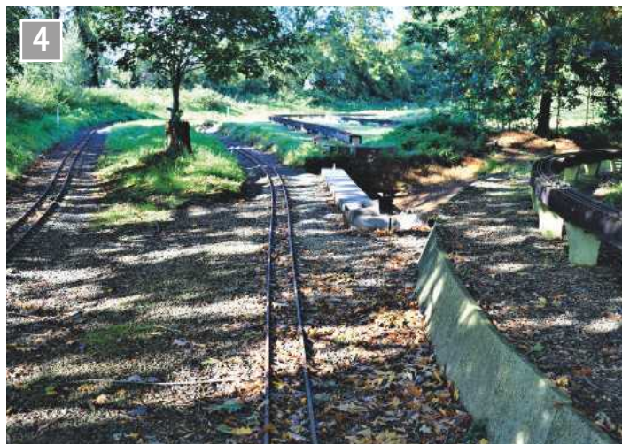
The connection point for the raised track, with the new track at the top and the existing on the right of the photo.
